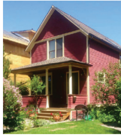
Potential municipal heritage resource home on 11A Street NW.
