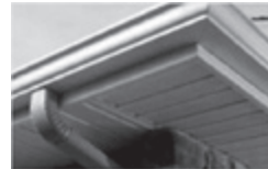
FASCIA, SOFFIT & EAVESTROUGH
