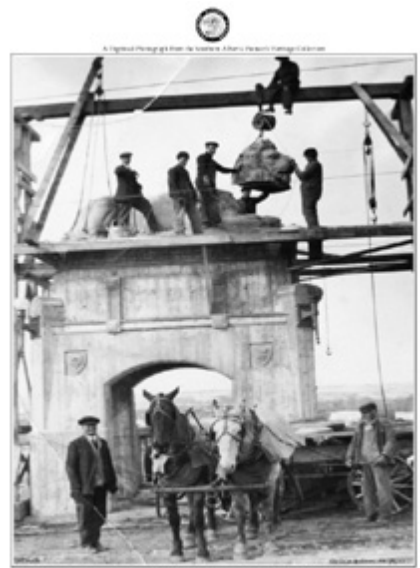
Calgary Herald, March 4, 1917. "Placing the Lion" at the Centre Street Bridge. Workmen place the lion on one of the four kiosks during the construction of the bridge. Lions were designed by James L. Thomson.
