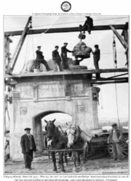
The installation of one of the Centre Street Lions in 1917. Image via the Southern Pioneer's Heritage Collection, pioneersalberta.org.
