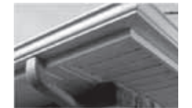
FASCIA, SOFFIT & EAVESTROUGH
