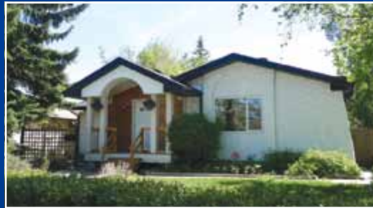
2207 PALISWOOD ROAD SW - $579,900
