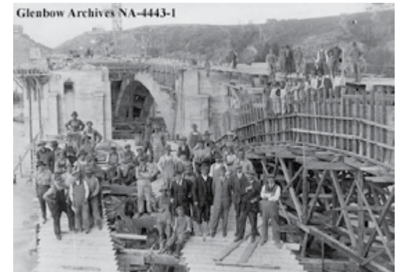
Workers on the bridge during its construction in 1916. Glenbow Archives
