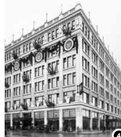
1. Edwardian commercial style building with a steel-and-concrete frame and terra cotta tile façade. The arcade (covered walkway) is supported by columns of Quebec granite and paved with terrazzo tiles.
